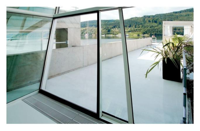
Automatic linear sliding door system for use on inclined glass façades
